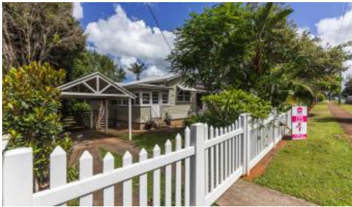
17A Green St, Alstonville
