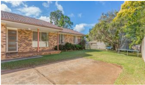
2, 50 Wardell Road, Alstonville
